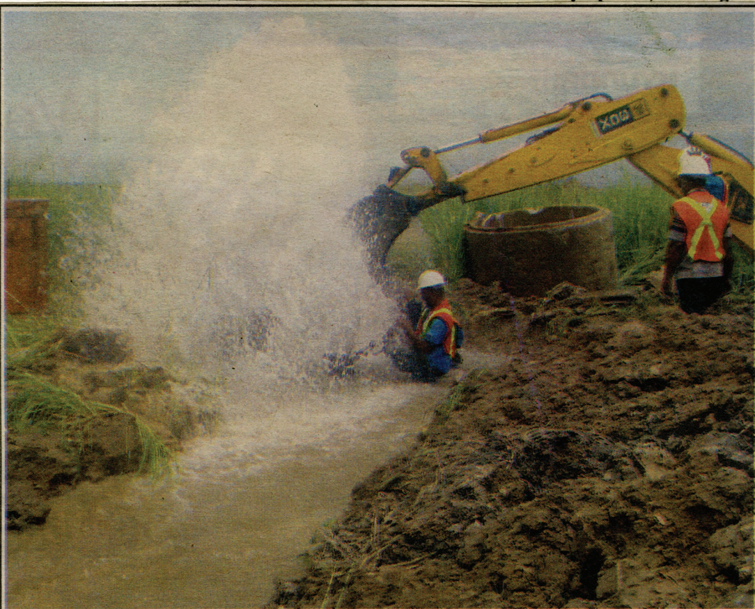
MASSIVE WASTE: Uncaring criminals caused over 200,000 persons in Central and South Trinidad to be deprived of water after they stole an air valve on Monday night, from this 54 inch water main at WASA's Caroni South Transmission Main in Chaguanas. This photo shows workmen repairing the gushing main where, according to WASA, 43 million gallons of drinking water were lost. SEE PAGE 13A
